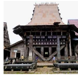
Figure 7 Traditional House of Bawamataluo Village
